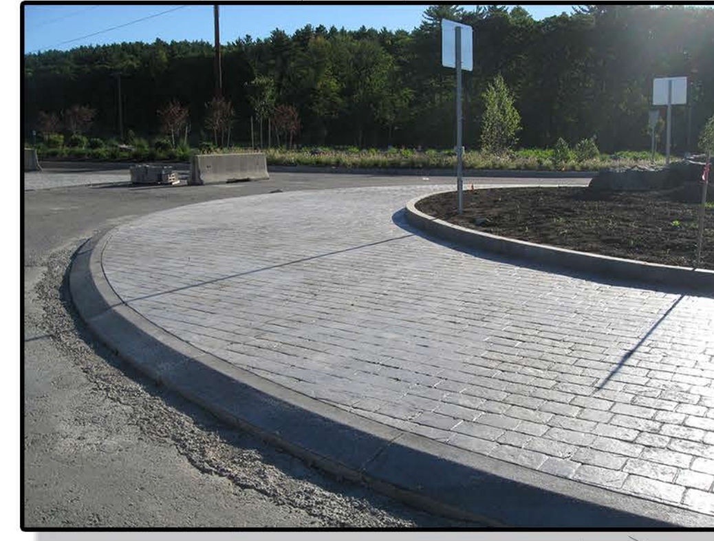
EXAMPLE OF STAMPED CONCRETE
